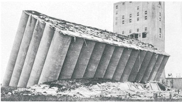
**Fig. 2.** The accident of the Transcona silo in Canada 1913 (taken from <http://www.archiseek.com/>).
